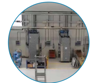
Lean Assembly stations for internal commissioning and FATs
